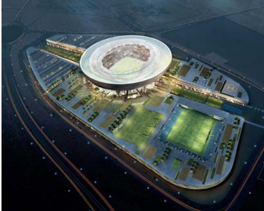
The 60,000 capacity stadium will be elevated and encased in a futuristic diagrid bowl
